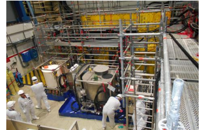
Chemical system decontamination preparatory works at CNT2
