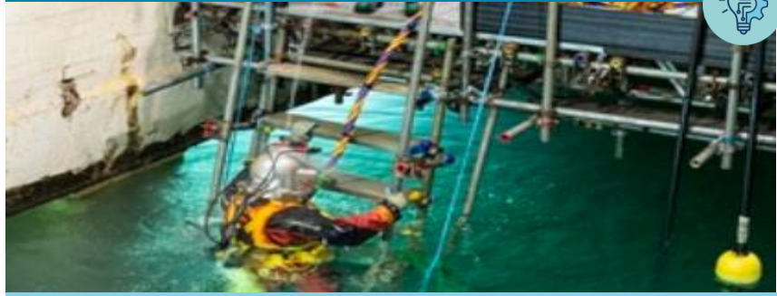
A diver going into the Pile Fuel Storage Pond on the Sellafield site
