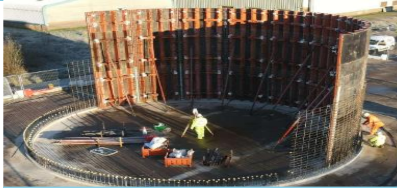
Pictured: 7.5 m high full-scale mock-up of the iconic Sellafield Pile Chimney barrel
